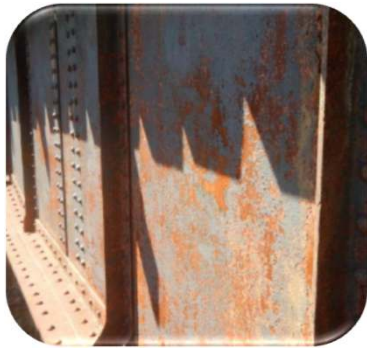
Surface coating failure
