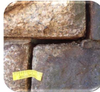
Missing masonry
