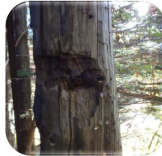
Cracked timbers
